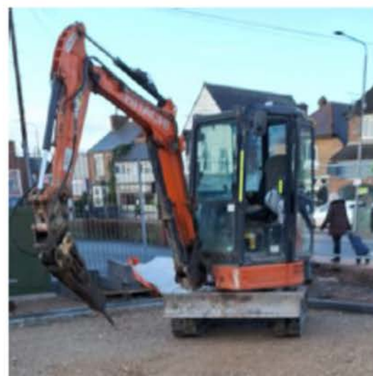
Image 2 – Plant left running with seatbelt plugged in.
